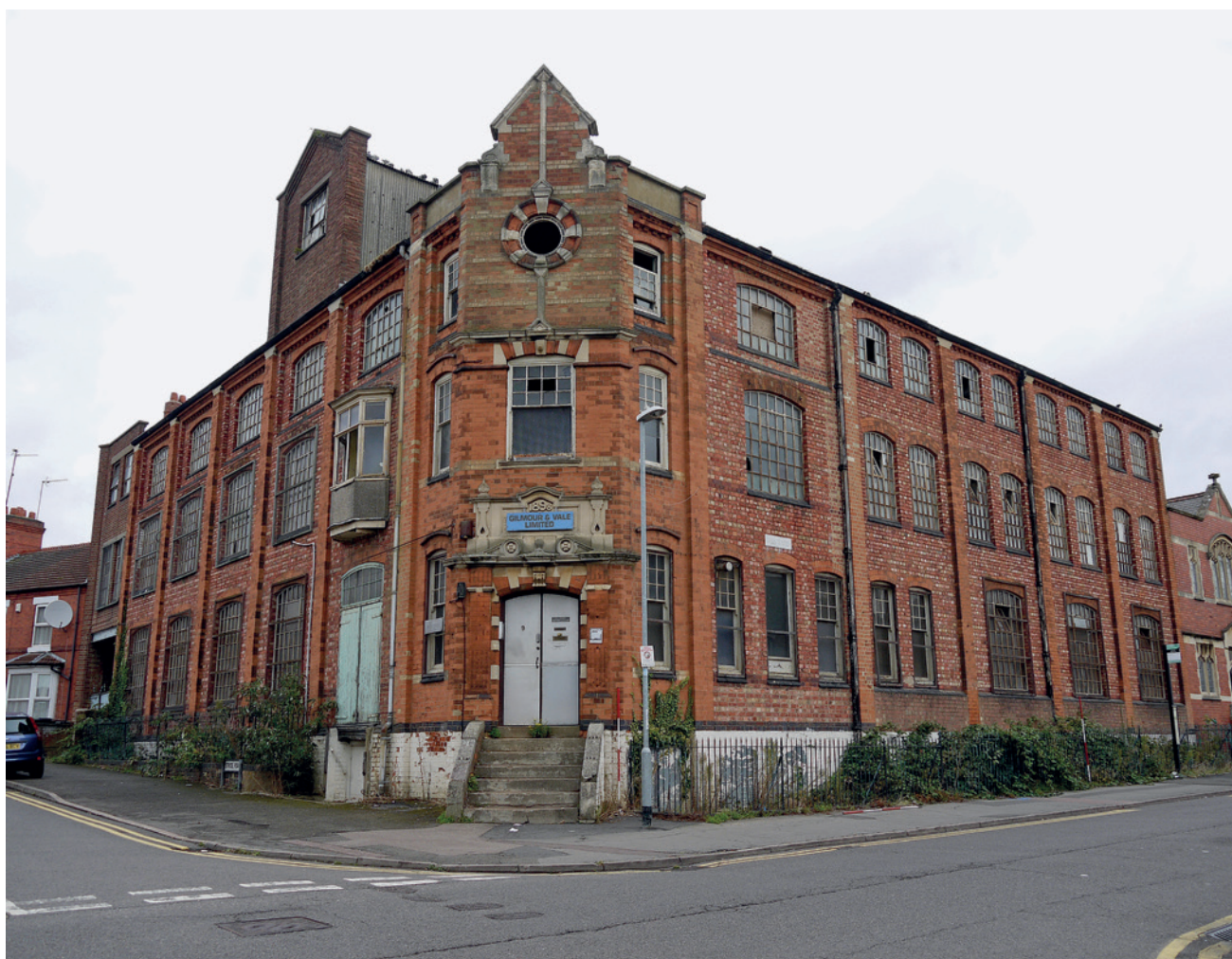
Figure 14: Wellingborough, The Former R. Rudlen & Co. Ltd.
