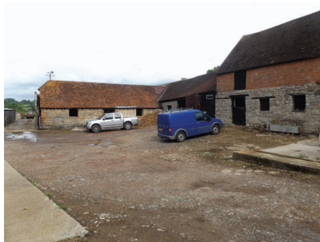
Figure 14: Preston Bissett, Church Farm buildings during conversion
