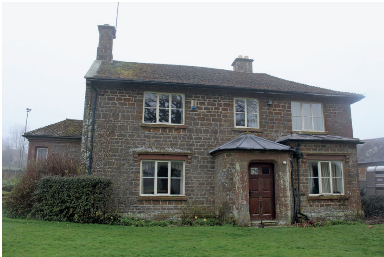
Figure 1: Hellidon, Leam House eastern elevation
