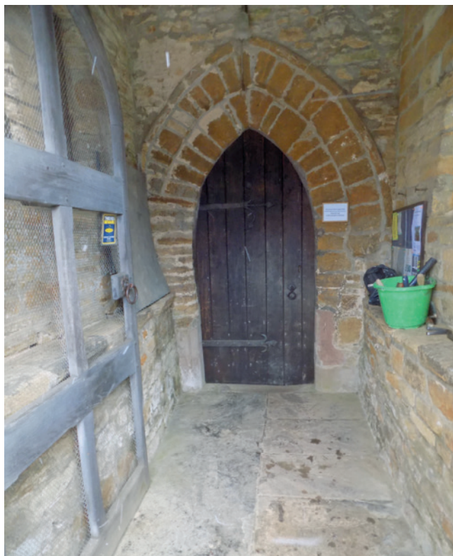
Figure 4: Badby Church porch before excavation, looking north
