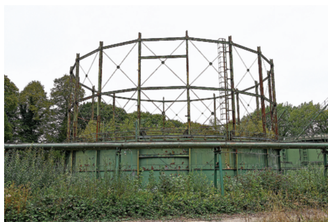
Figure 19: Denham, General view of 1926 frame-guided Gasholder
