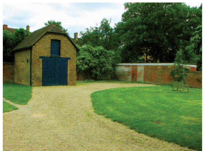
Figure 3: Former stable complexes at 62 (right) and 64 (left) Banbury Road, Oxford
